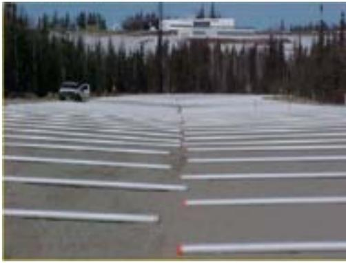
Hairpin thermosyphons being put in place during construction of Thompson Drive on the UAF campus. Each thermosyphon helps to keep the permafrost below remain frozen. Thompson Drive is a stop on the permafrost tour.
