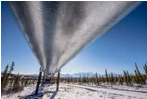
The Trans-Alaska Pipeline is one of the world's engineering marvels. The 48-inch diameter pipeline navigates through three major mountain ranges and over 800 miles from Prudhoe Bay to Valdez. The pipeline viewpoint is a stop on the permafrost tour.
