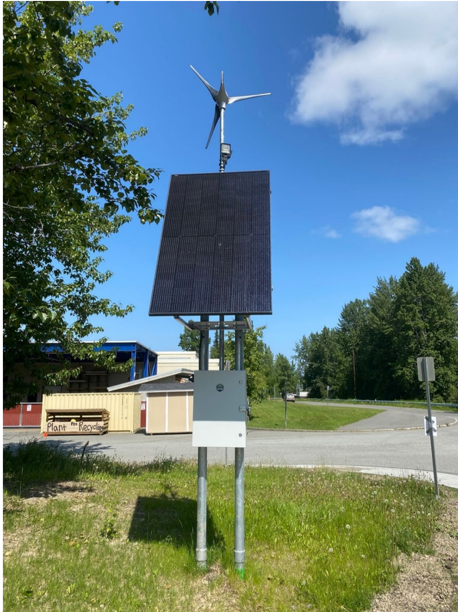
Figure 5-1 The smart light unit at UAA campus
