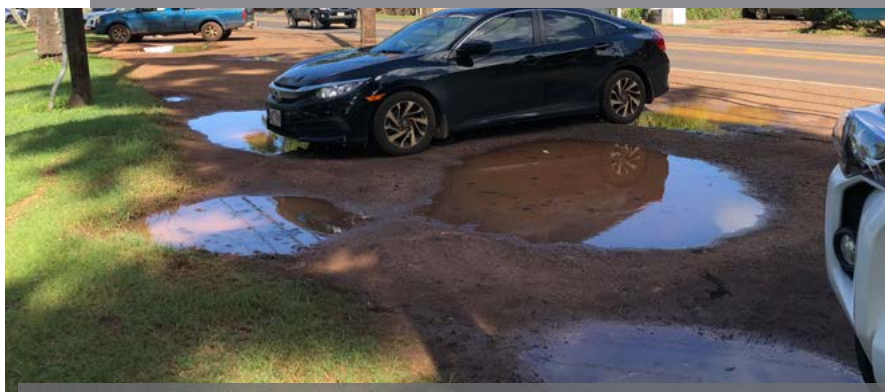
Flooded Parking on the North Shore of Oahu, Hawai'i, November 18, 2018. Photo by Suwan Shen.
