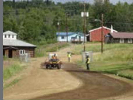
Dust palliative being spread on a road in Ruby, Alaska.
