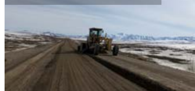
A grader evens the wearing surface of the Dalton Highway, Alaska during spring melt.
