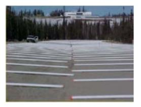
Hairpin thermosyphons being put in place during construction of Thompson Drive on the UAF campus. Each thermosyphon helps to keep the permafrost below remain frozen. Thompson Drive is a stop on the permafrost tour.
