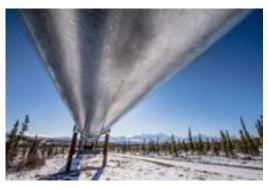
The Trans-Alaska Pipeline is one of the world's engineering marvels. The 48-inch diameter pipeline navigates through three major mountain ranges and over 800 miles from Prudhoe Bay to Valdez. The pipeline viewpoint is a stop on the permafrost tour.
